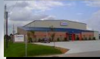
Houston Service Center Turnarounds, Repair; Actuator Assembly Houston, Texas
